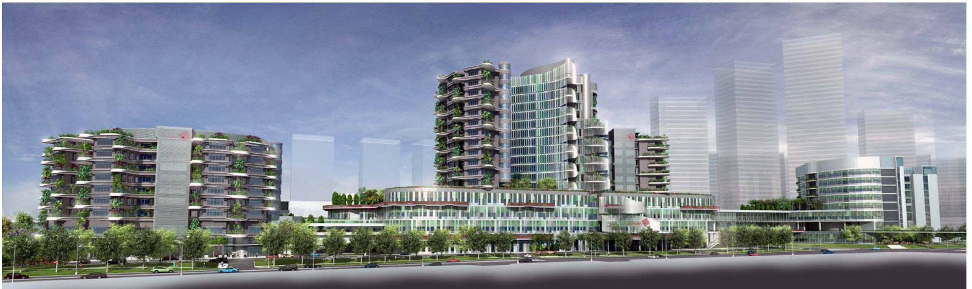
< Singapore, Ng Teng Fong Hospital Project >
